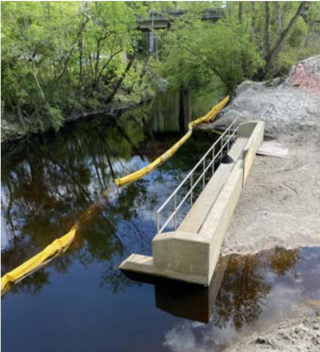
**BLACK CREEK INLET FACILITY:** The steel sheets separating the creek from the inlet facility construction have been removed. The inlet grates, seen in last month's newsletter, are completely covered indicating that at this level, there is sufficient water in the creek for pumping to take place.
