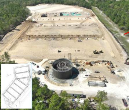
**TREATMENT AREA:** The pre-stressed concrete water tank was still under construction when this aerial was taken. It will hold water from the pipeline for distribution to the treatment ponds. In the top photo, some of the waterproof liner for the treatment ponds is seen with the now completed water tank in the background. Treatment cells, No. 1 to 3 are scheduled for start-up and testing in November 2024. Cells No. 4 to 6 will follow in February, 2025.
