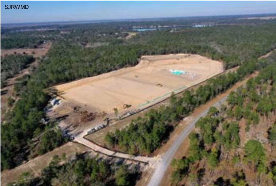
**TREATMENT AREA:** Construction of the treatment ponds is proceeding. Blue PVC pipe, fittings and concrete water structures can be seen on site. As seen in this photo, the nearest treatment ponds are No's 1, 2 & 3. They will be completed and be on line at the end of 2024. Treatment ponds 4, 5 & 6 are scheduled for completion in 2025.
