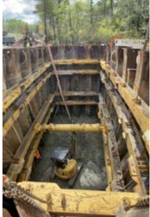
Inlet site by the SR16 Bridge at Black Creek: Top right photo shows the sheet pile where the intake will be located at the creek's edge. The lower right photo shows inside the pit being dug out from which the pipe line will be horizontally "micro tunneled" to the pump station pit.
