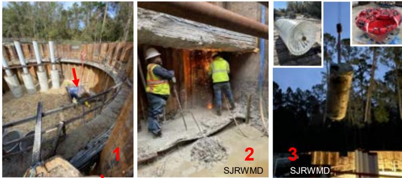
**A PROJECT MILESTONE:** With heavy rain predicted for 12/16/23 and the flooding of Black Creek forecast, workers in the pit (1) at the lowest level under the pump station, worked urgently to cut a hole through the 1/2" sheet steel (2) allowing the micro tunneling machine (3) to be withdrawn from the conduit.
