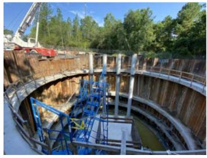
**BLACK CREEK PROJECT PUMP STATION SITE:** 6/26/2023. Left photo shows the pipes leading to the future pumps in the pumphouse. The foundations have been poured. Workers are constructing the rebar cages to be fastened to the foundation's steel bars. In the middle photo are precast pipes that will be placed over the pipes/rebar and filled with concrete. On right, the pumps work to keep up with rainfall.
