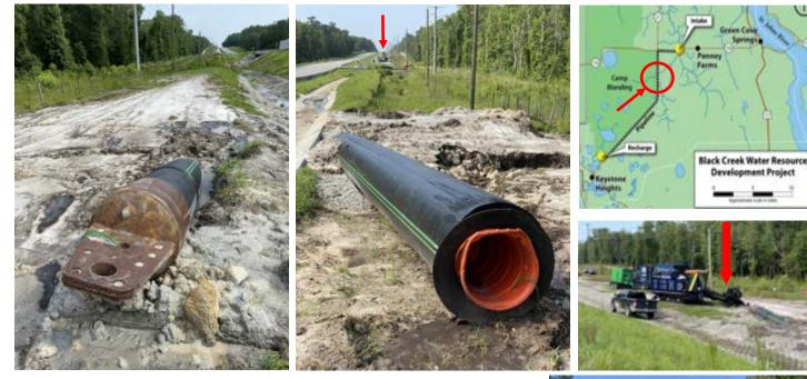
**HORIZONTAL BORING UNDER CREEK COMPLETED:** As located in the red circle in the map in the upper right, this portion of the South Prong of Black Creek has its origin in Camp Blanding and crosses under SR-21. By boring, the pipeline project, as it continues south in the SR-21 right-of-way, will have no impact on the creek. A 1,600 ft tunnel was bored. At the terminal end, the cutting head removed and a fitting attached to the HDPE Pipe. The 30" pipe was drawn back through the tunnel and out at
